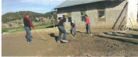
Clearing out the land for the slab
